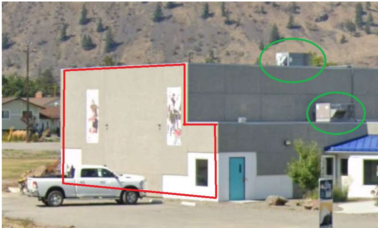
Figure 6: Proposed solar air heating application: collector mounted on red indicated wall face, preheats air from green indicated RTUs
